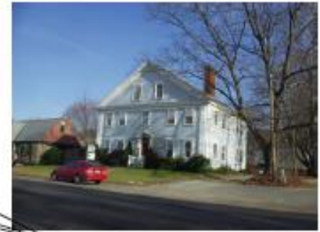
12 units of Housing in Town House type structures
