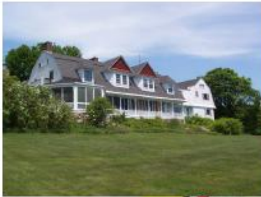
16 units of Extended Care Housing in a traditional home style
