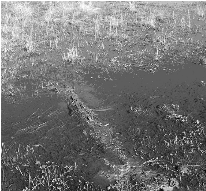
Figure 10. Bundle of cottonwood cuttings placed in a small ditch to slow run off and ultimately generate riparian vegetation through hardwood cutting. Photo by Rick Barney, NRCS
