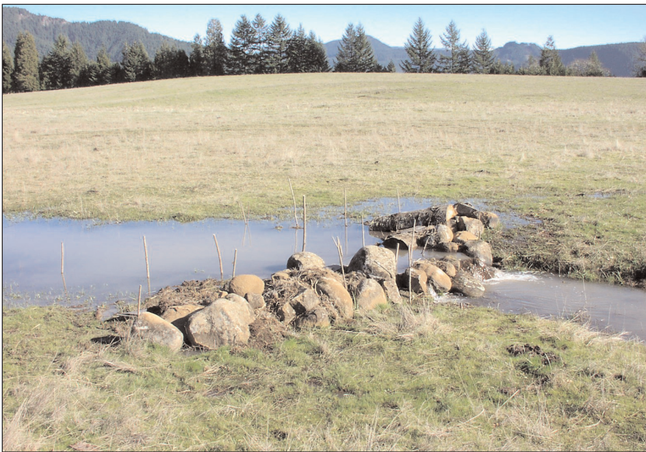
Figure 8. A low dirt berm reinforced with rock. Notice willow cuttings in place upstream of the berm. Photo by Rick Barney, NRCS.
