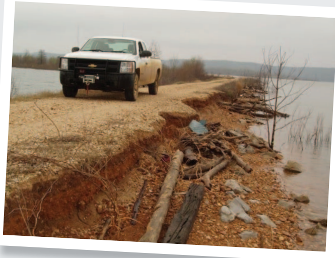
Levee restoration, Tennessee NWR, TN | FWS
