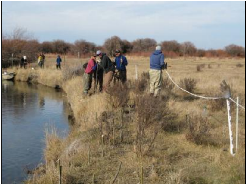
Fencing to exclude uncontrolled cattle-grazing and restore riparian vegetation Photos courtesy of Teton Regional Land Trust
