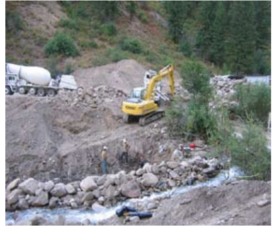
Restoring habitat by repairing fish culverts
