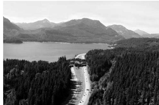
Simulation of overpass to be built for the Snoqualmie Pass East I-90 Project in Washington
