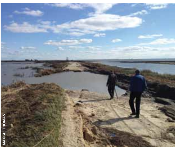
Hurricane Sandy hammered coastal refuges such as Edwin B. Forsythe in New Jersey. From the dikes and roads that have been severely damaged to the wetlands that are now littered with debris from homes and boats, the storm caused millions in damages to the Refuge System.
