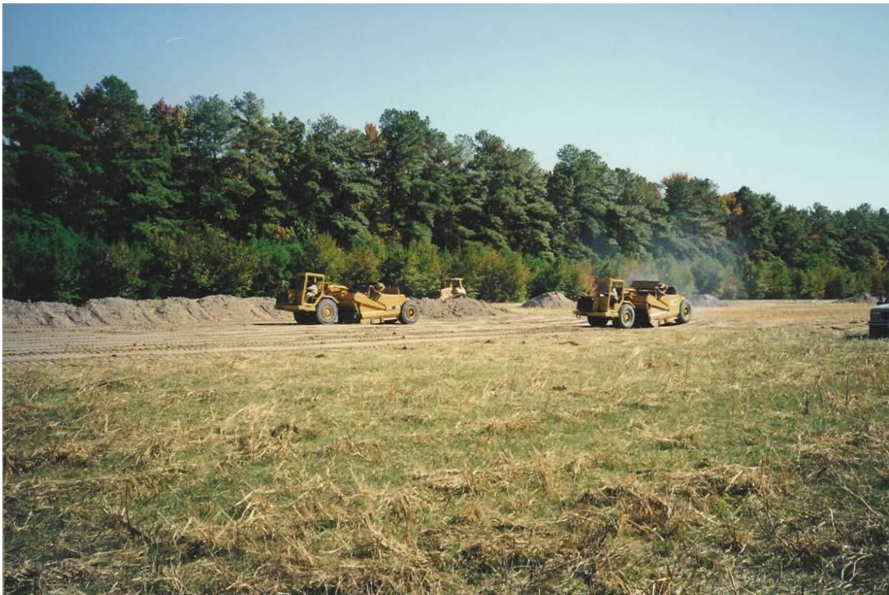
Constructing the wetlands.
