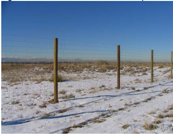
Figure 5c. Proposed woven wire perimeter fence.
