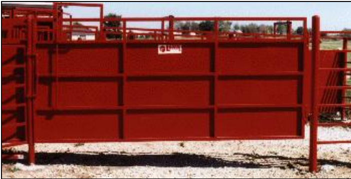
Figure 7. A bison gate with solid sheet of steel attached.
