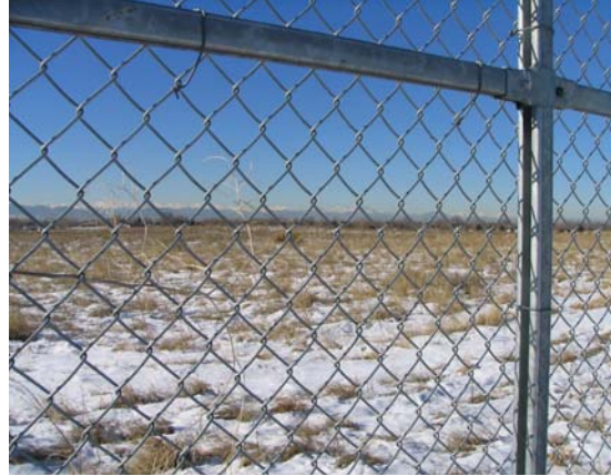
Figure 5b. Current Fence Close-up.
