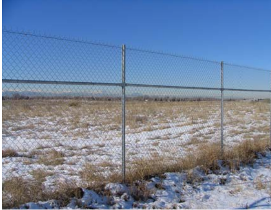
Figure 5a. Current RMANWR chain-link perimeter fence.
