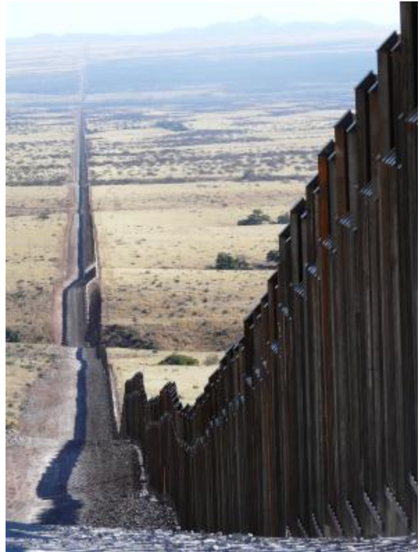
A border wall and patrol road slice across a National Park and a National Conservation Area. Photo: Matt Clark
