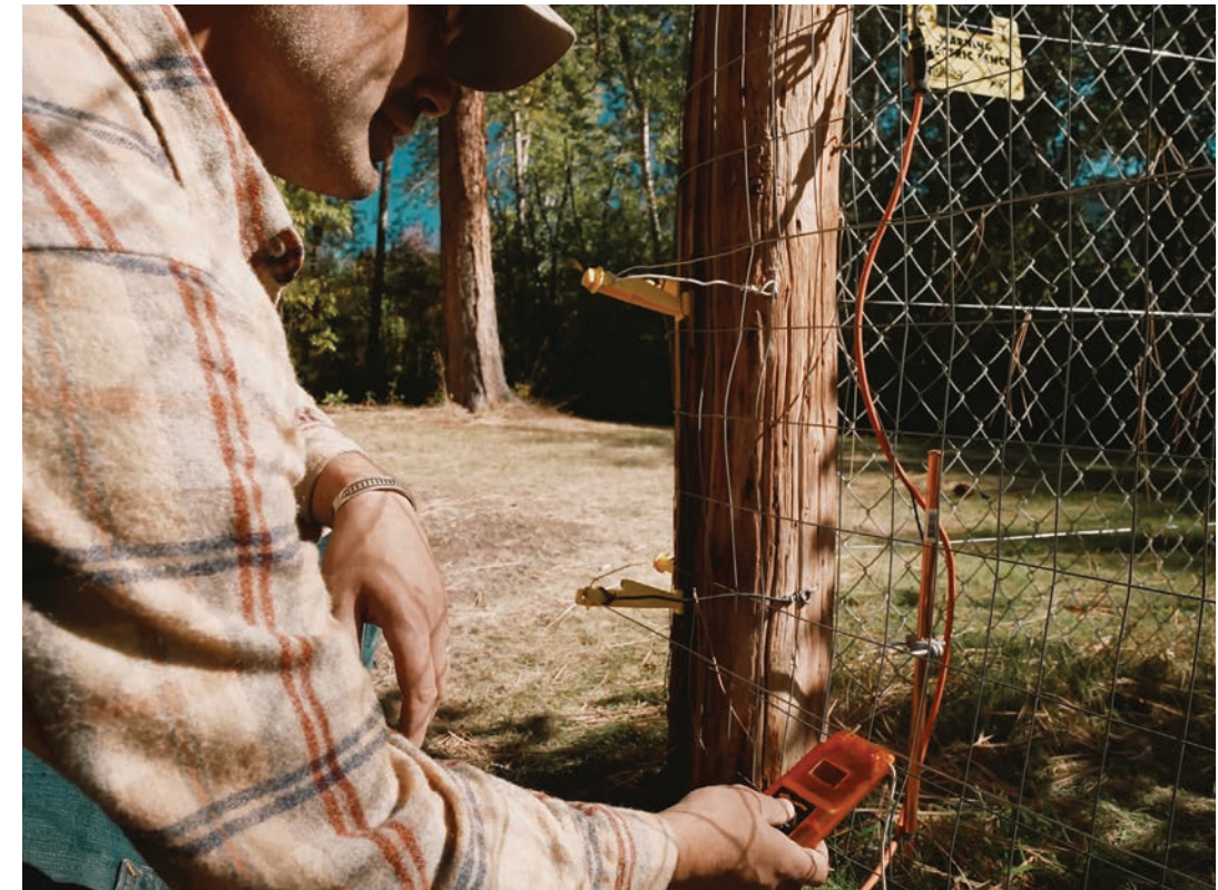
Russ Talmo, Rockies and Plains associate at Defenders of Wildlife, installs an electric fence to deter grizzly bear activity from private property.
